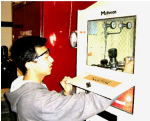
Smaller access door (shown above) should be used to turn on gas cylinder valve rather than the larger door which was opened.
