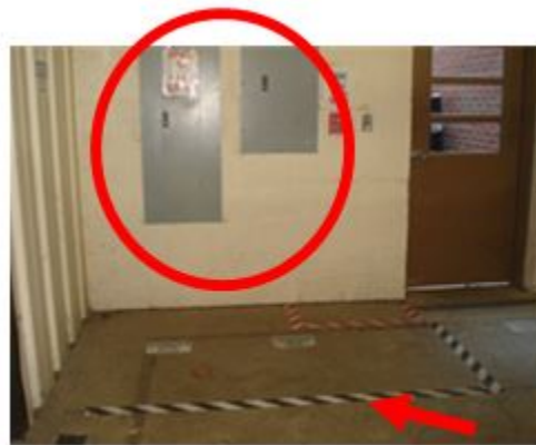
Building's Electrical Service Panels are taped off to keep free from obstructions.
